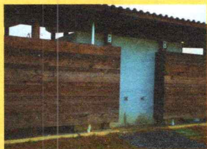
Shower houses at the Summit are built of locally harvested lumber.
